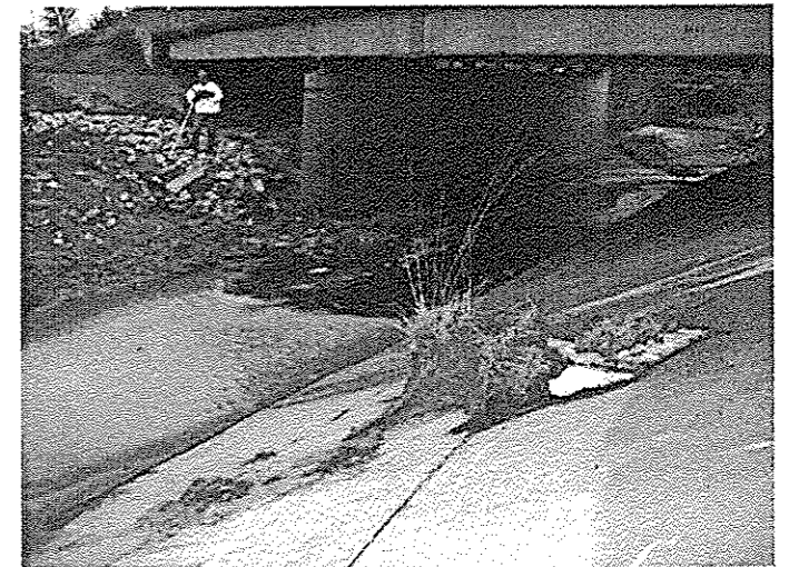
ELEVATION VIEW ⑧ (Looking West)
