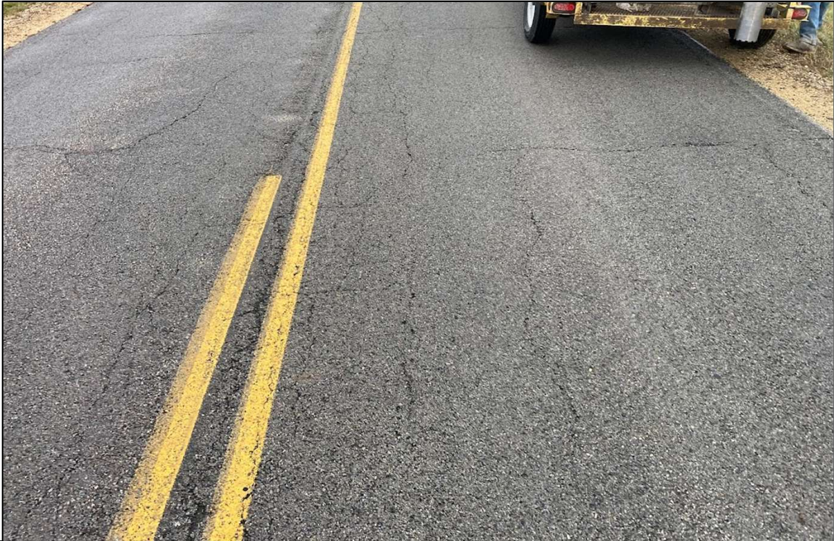
Existing Roadway Condition
