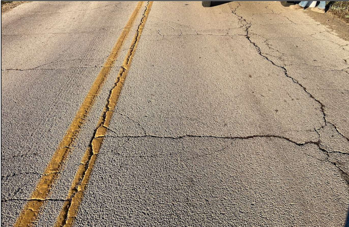
Existing Roadway Condition
