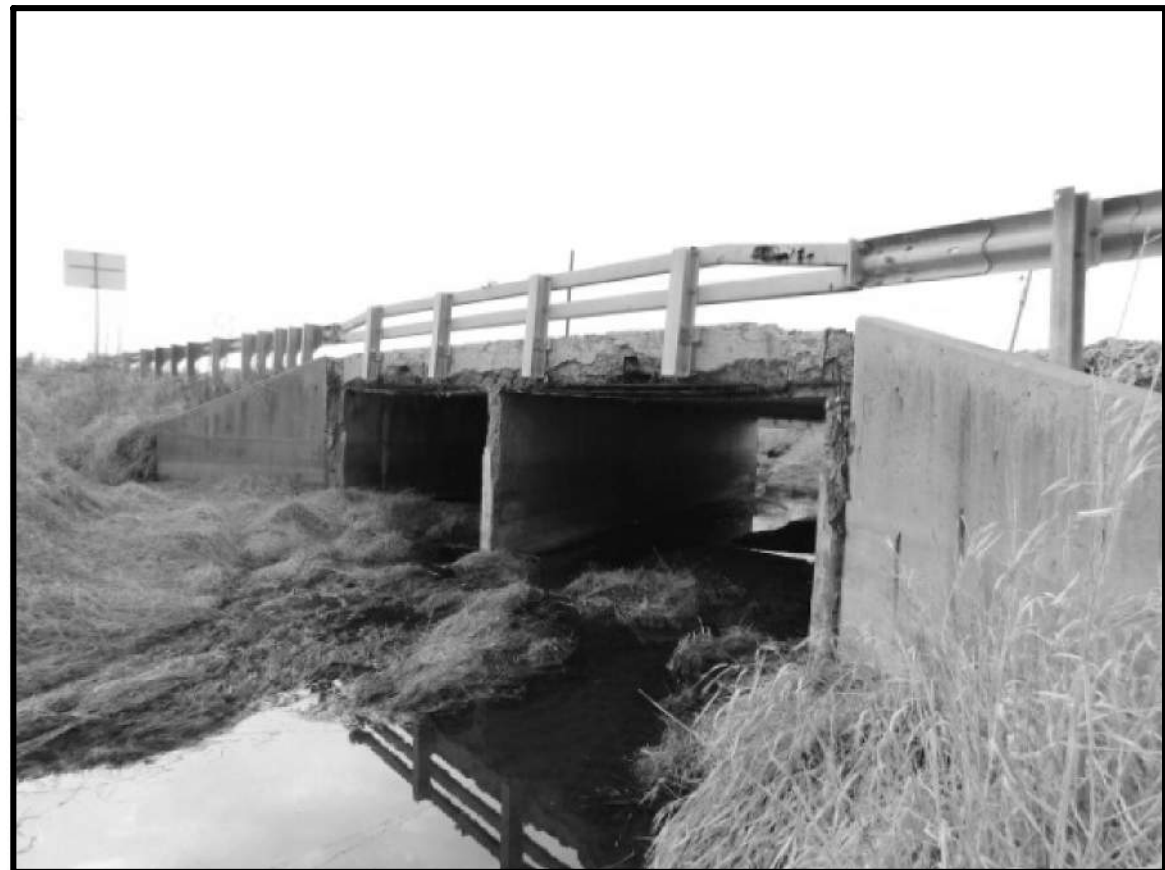
PHOTO SHOWING SOUTH SIDE OF CULVERT
