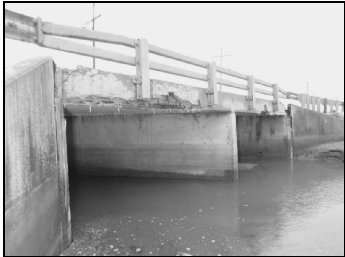
PHOTO SHOWING NORTH SIDE OF CULVERT
