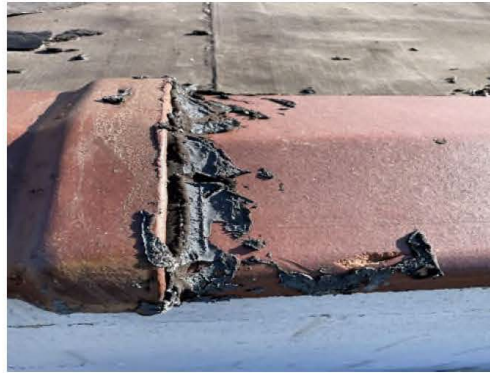
HA-10: Black Roof Coping Tile Sealant
