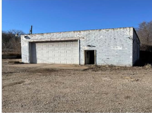
View of Building – Rear
