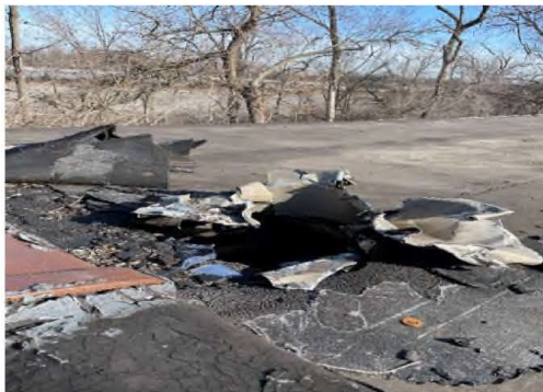
HA-11: Black Built-Up Tar/Tar Paper Roof
