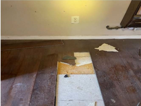
HA-1: Brown Laminate Flooring HA-2: Gray 12" x 12" Vinyl Floor Tile and Yellow Mastic
