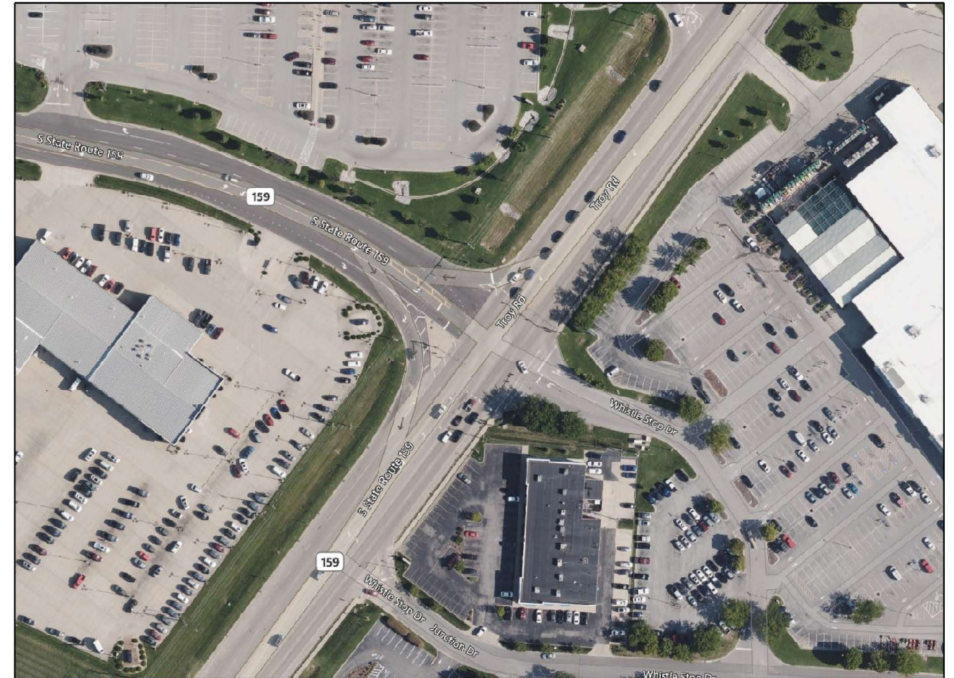
LOCATION # 20 IL 159 @ TROY RD. - EDWARDSVILLE INTERSECTION ID # 4362
