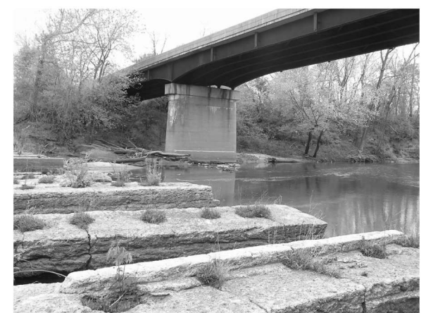
PIER 2 (Looking Southeast)
