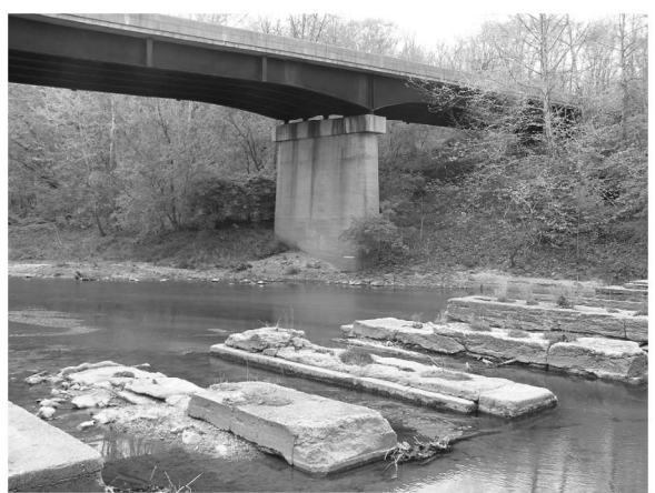
PIER 1 (Looking Southwest)
