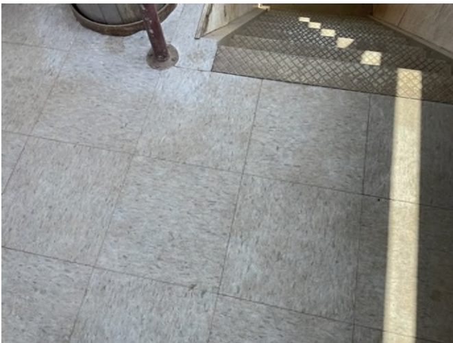
HA-5: Gray 12 x 12 Floor Tile HA-6: Yellow Floor Tile Mastic
