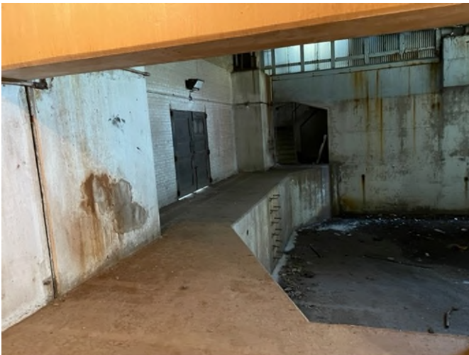
HA-3: Gray Concrete Foundation and Walls
