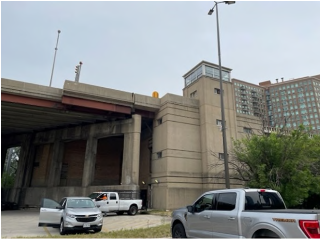
View of the Southwest Bridge Tender House
