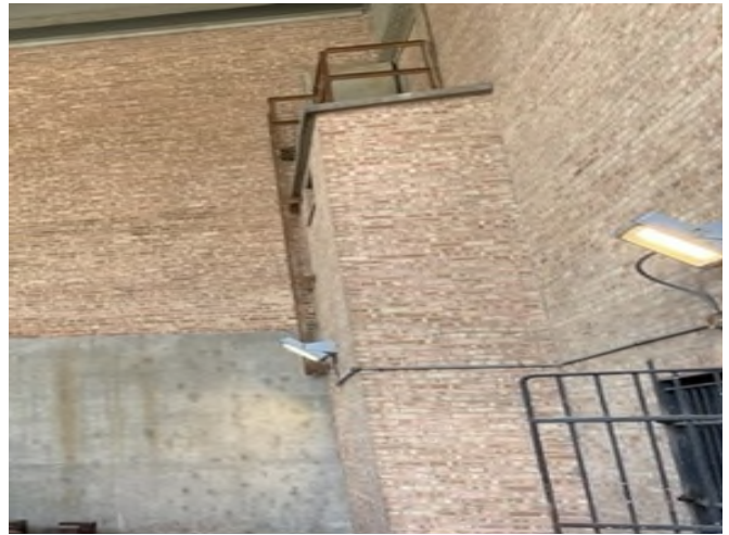
HA-1: Red Exterior Brick HA-2: Gray Mortar
