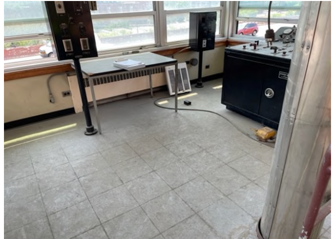
HA-9: Yellow Cove Base Mastic
