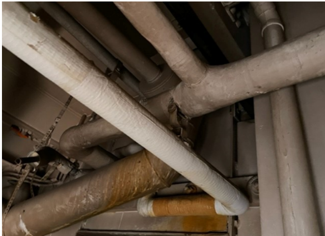
HA-10: White Air Cell Pipe Insulation
