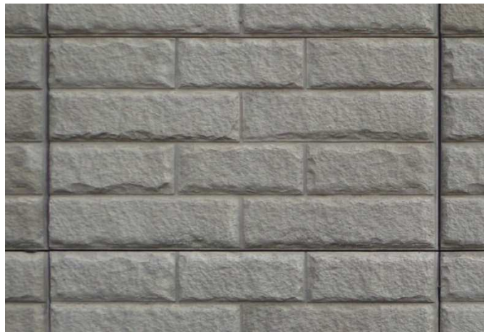
Exhibit C- Gravity Type Precast concrete Units Pattern
