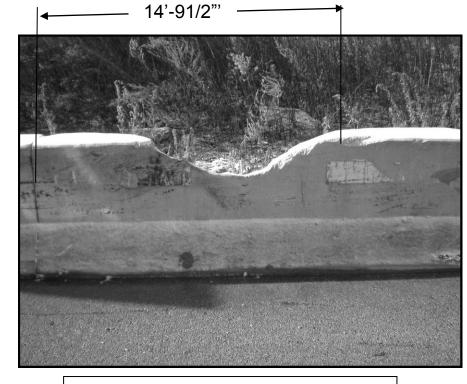
PARTIAL DEPTH BARRIER REPAIR FOR MORE DETAILS SEE SHEET # 9
