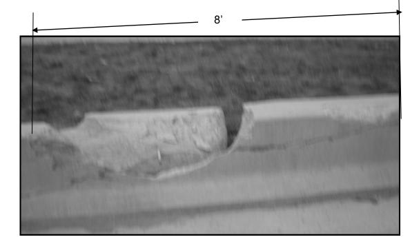
**FULL DEPTH REPAIR** REPLACE 8 FT OF BARRIER WALL FOR MORE DETAILS SEE SHEET #8
