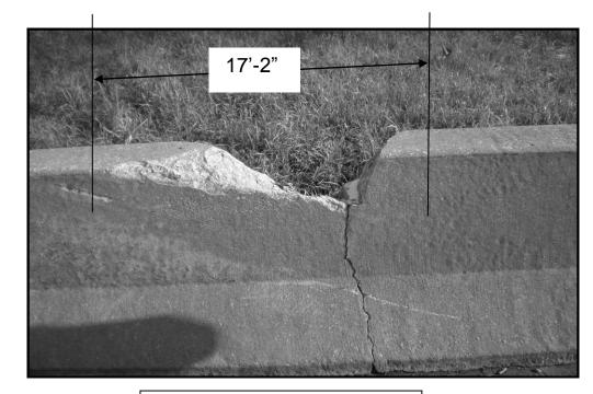
FULL DEPTH REPAIR REPLACE 17'-2" OF BARRIER WALL FOR MORE DETAILS SEE SHEET # 8
