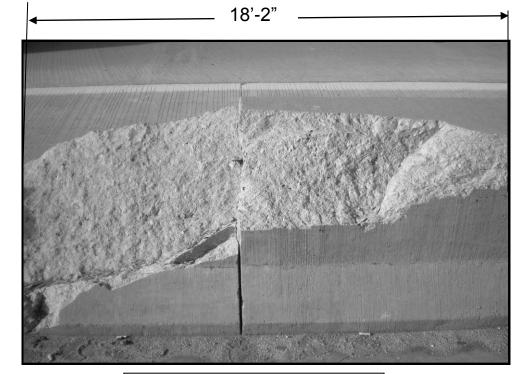
**FULL DEPTH REPAIR** REPLACE 18'-2" OF BARRIER WALL FOR MORE DETAILS SEE SHEET #8
