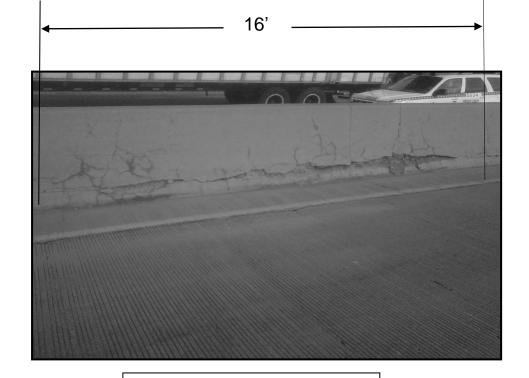
**FULL DEPTH REPAIR** REPLACE 16 FT OF BARRIER WALL FOR MORE DETAILS SEE SHEET #8
