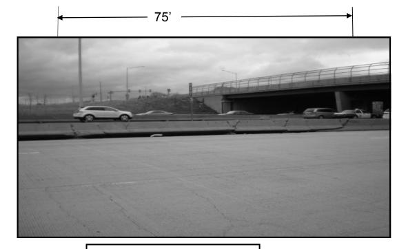
FULL DEPTH REPAIR REPLACE 75' OF BARRIER WALL FOR MORE DETAILS SEE SHEET #8
