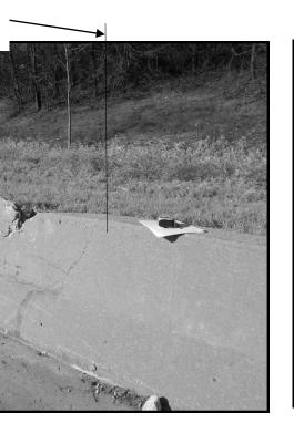
**FULL DEPTH REPAIR** REPLACE 12 FT OF BARRIER WALL FOR MORE DETAILS SEE SHEET #8
