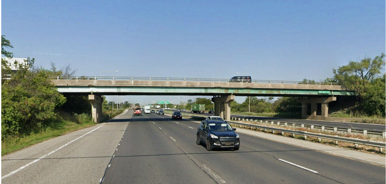
Exhibit 2a – Existing Bridge, Looking East
