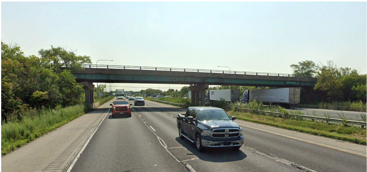
Exhibit 2b – Existing Bridge, Looking West
