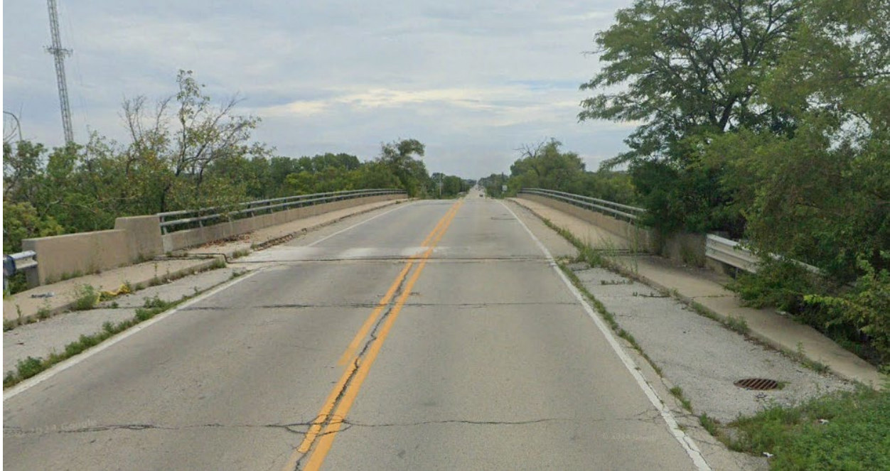
Exhibit 2c – Existing Bridge Deck, Looking North
