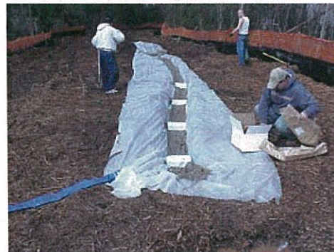
4) Place Floc Logs (upstream end)
