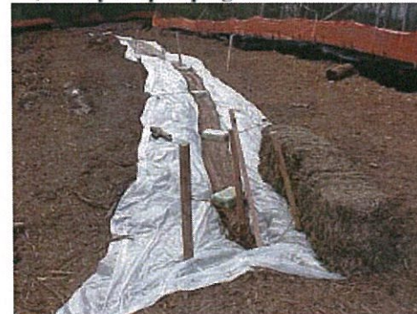
6) Ready for pumping
