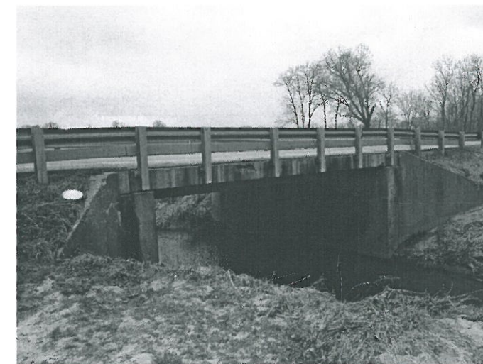
ELEVATION VIEW (7) (Looking Southwest)
