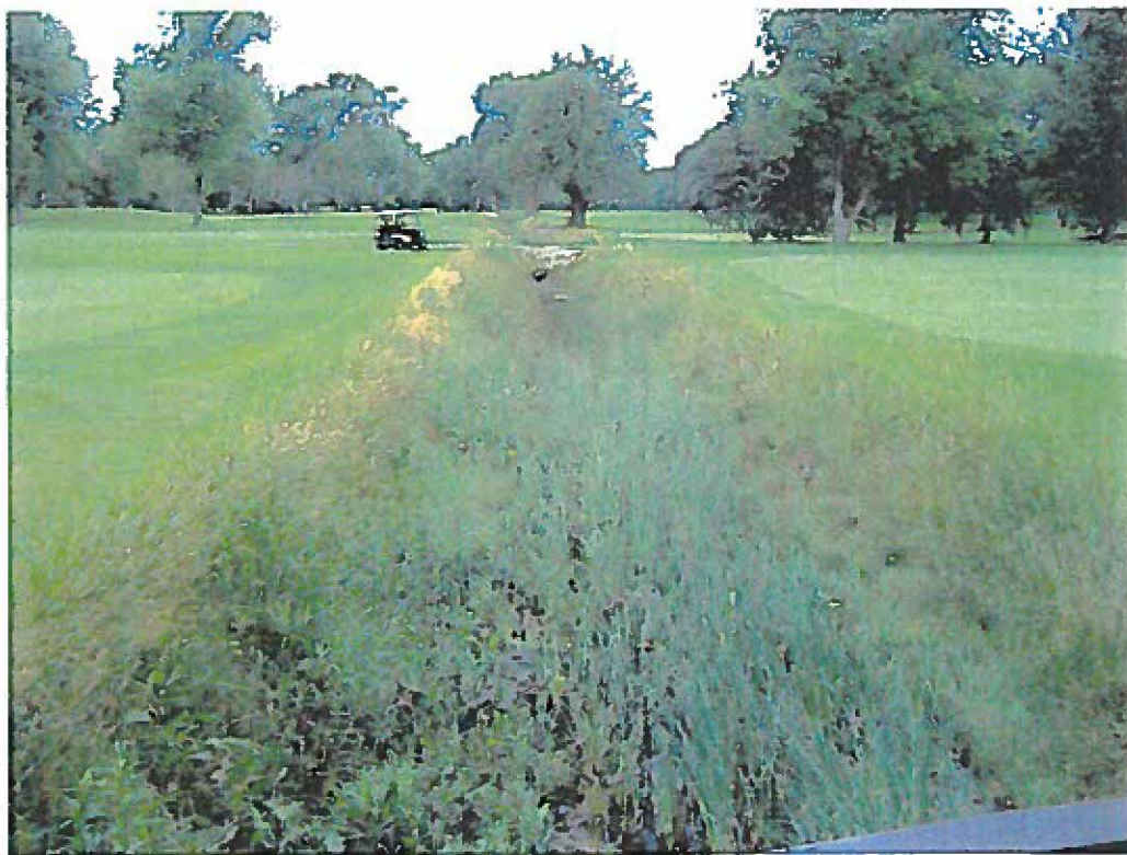
Downstream View of Unnamed Tributary from Wooden Bridge
