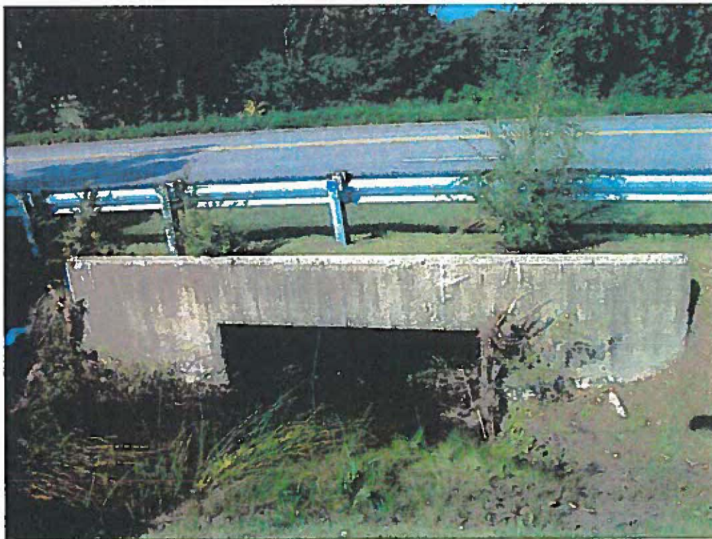
Existing 3'x8' Box Culvert (Upstream View)
