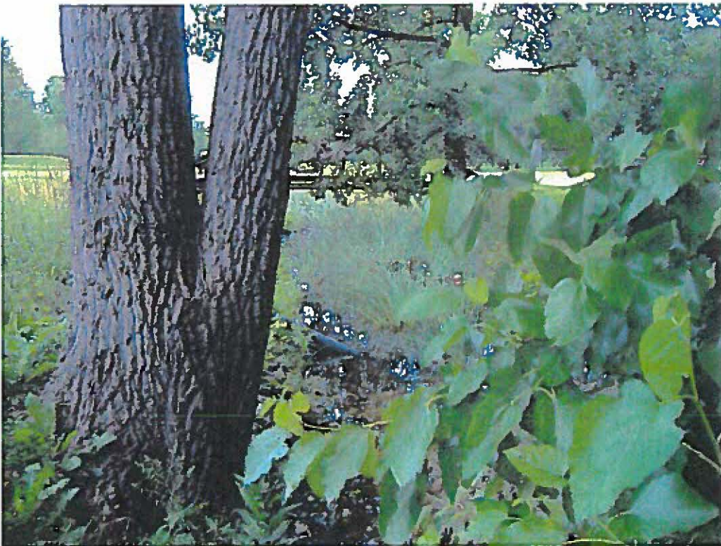
Downstream View of Unnamed Tributary from Dixie Highway Culvert
