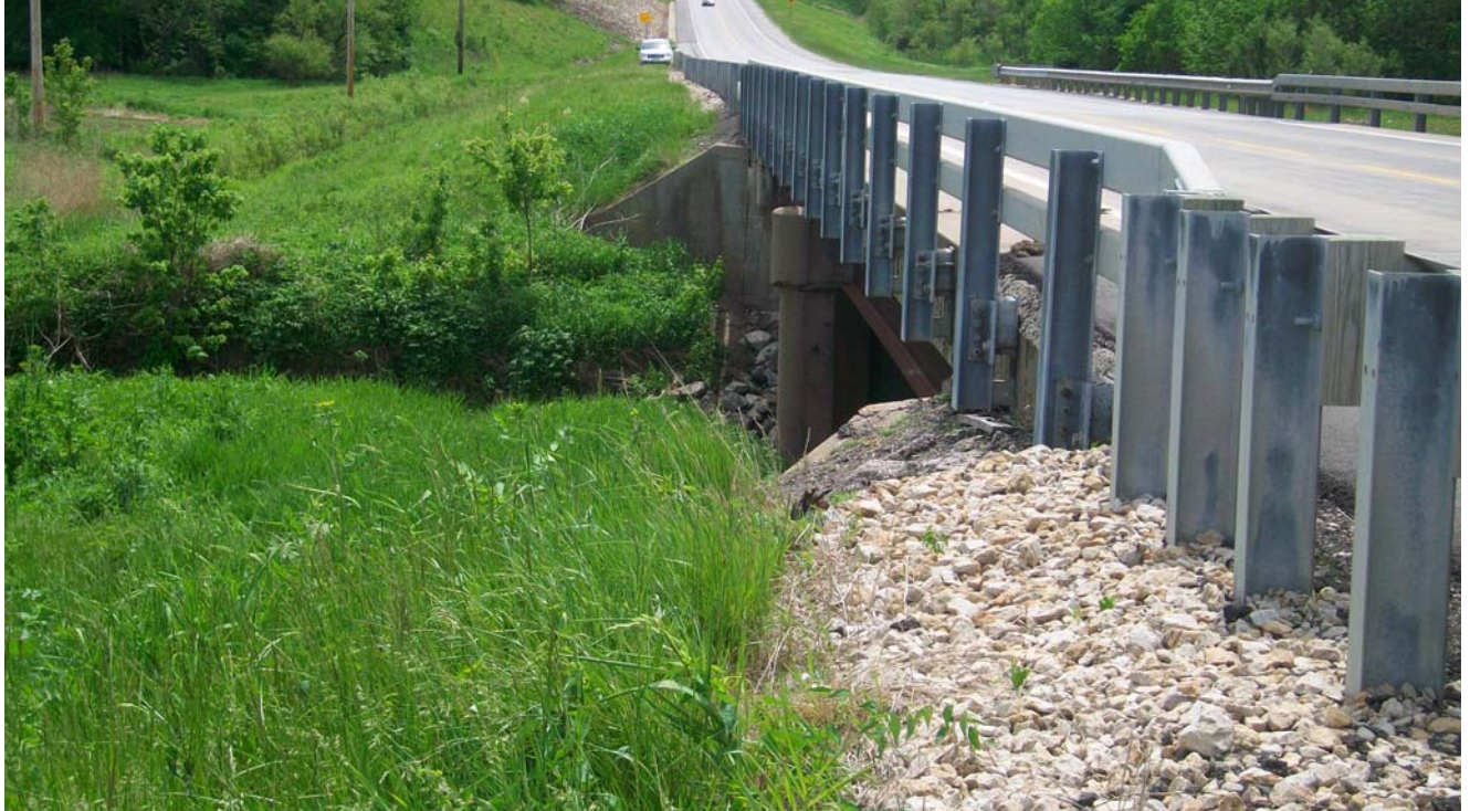
Picture # 7 Southeast ditch
