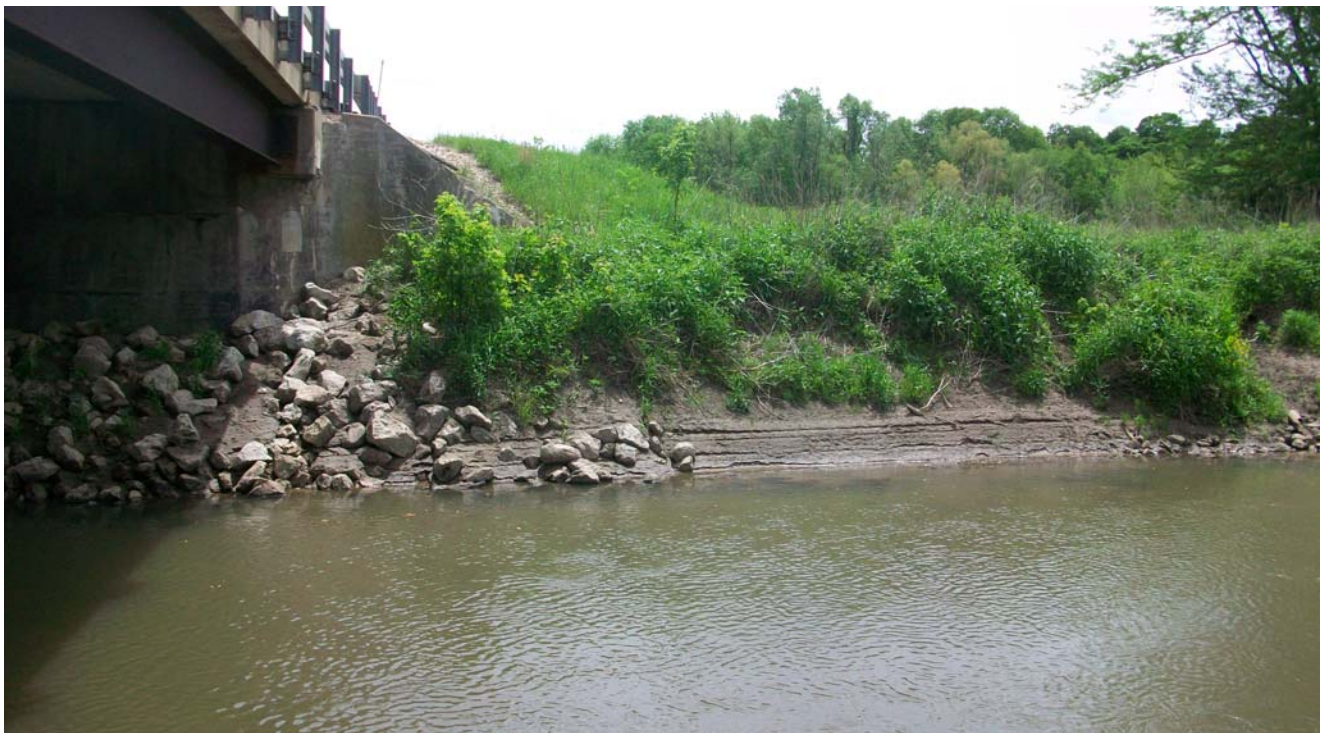
Picture # 6 Southwest creek bank
