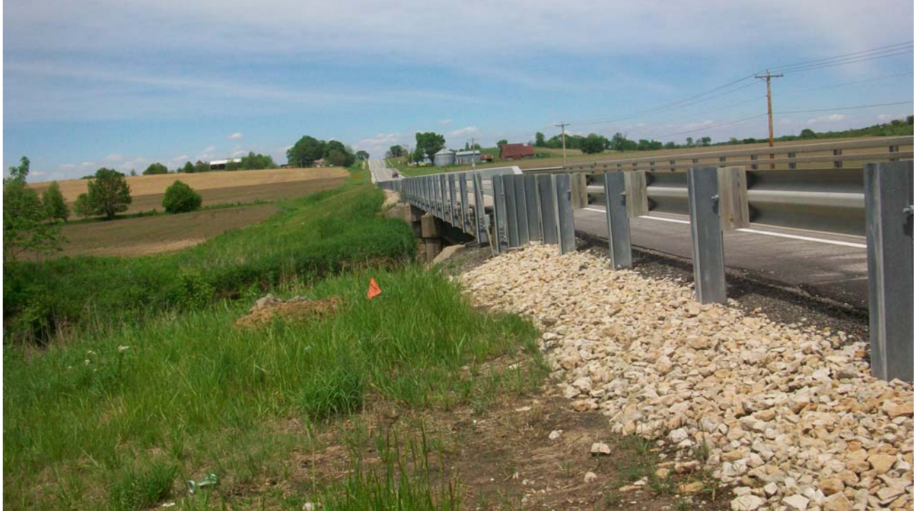
Picture # 5 Southwest ditch
