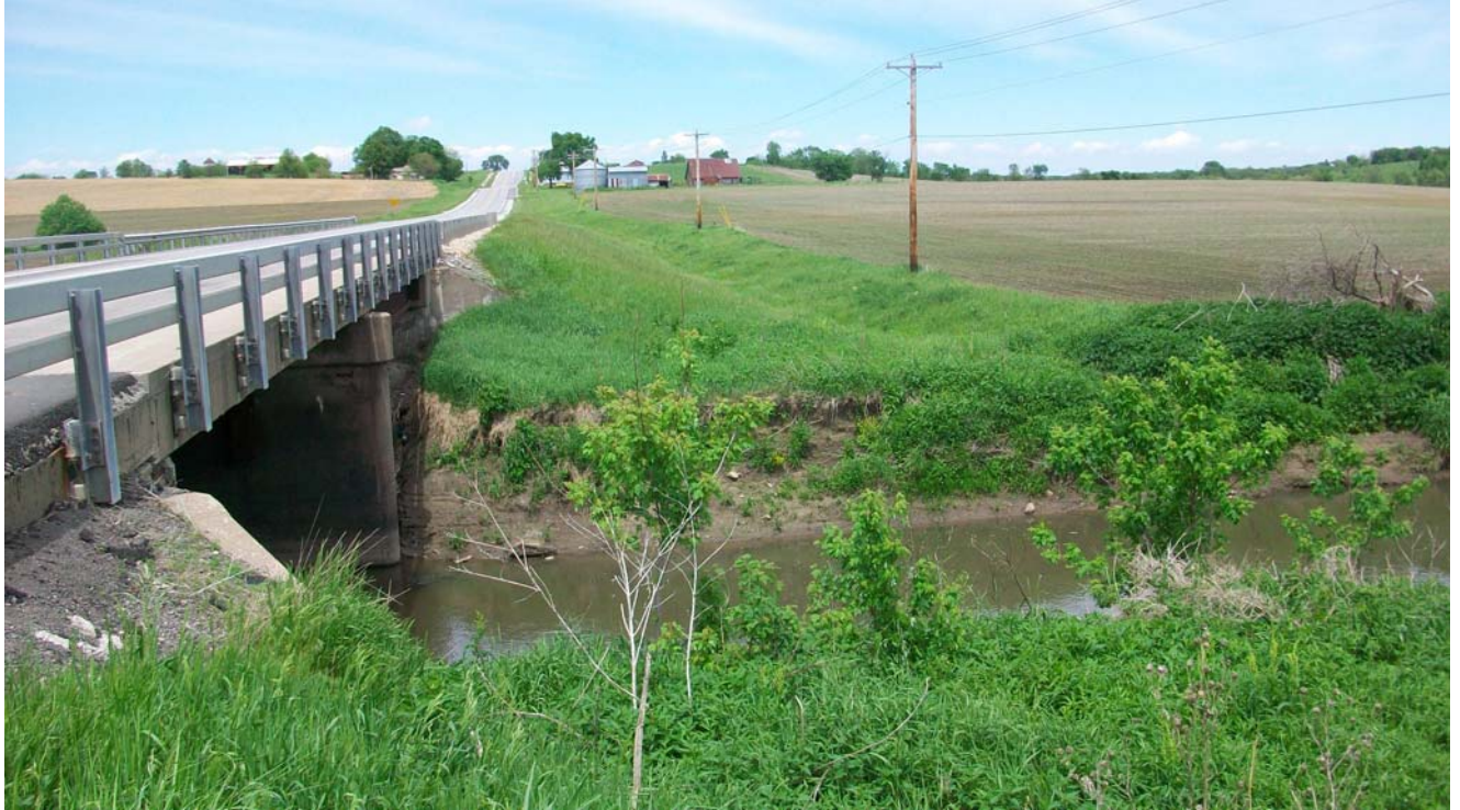
Picture # 3 Northeast ditch
