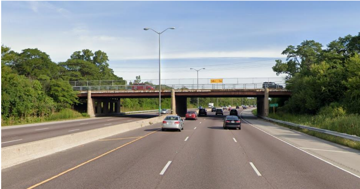
Exhibit 2 – Oakton Street Bridge Looking North on I-94
