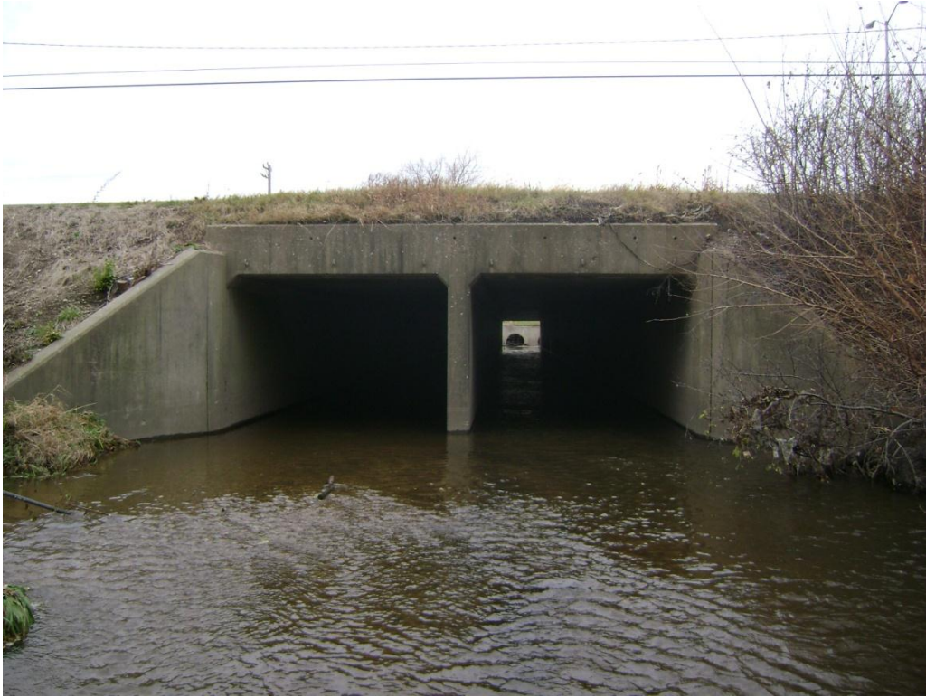
Downstream face of I-294
