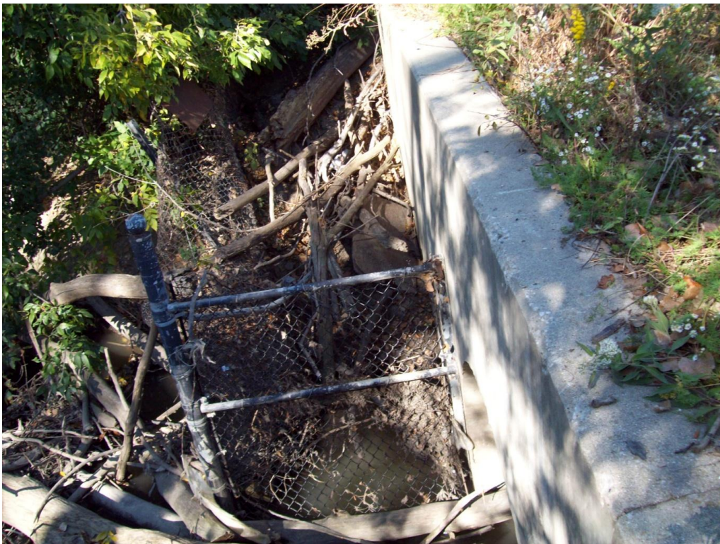
Looking at north bank of County Line Road from headwall
