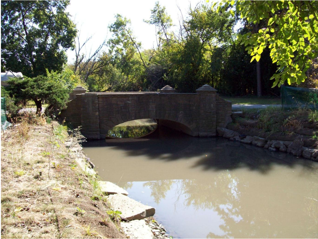
Upstream face of Cemetery Road #1 bridge
