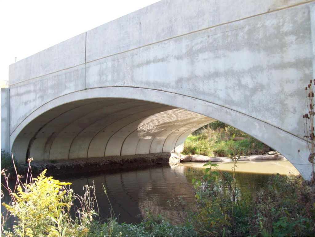
Upstream face of Industrial Access Road from west bank
