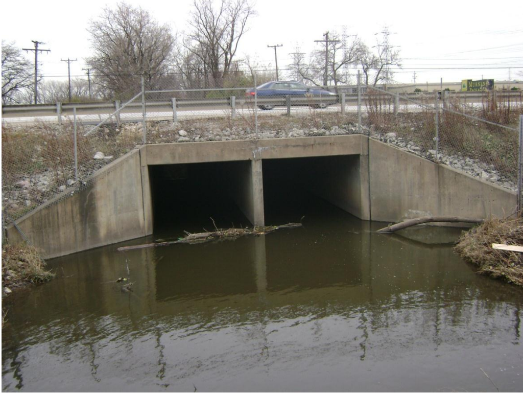
Upstream face of I-294
