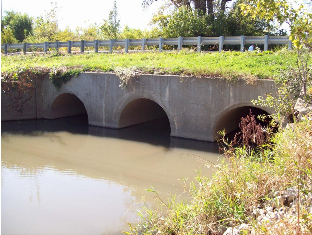
Downstream face of County Line Road from north bank
