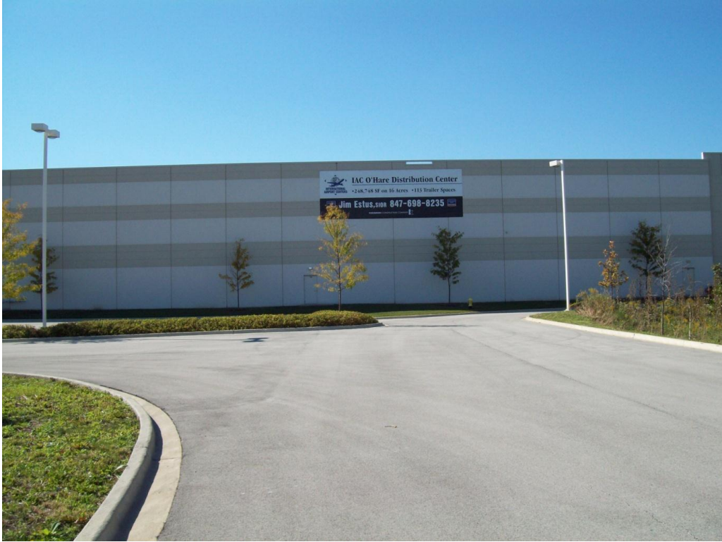
Industrial Access Road looking west at industrial building
