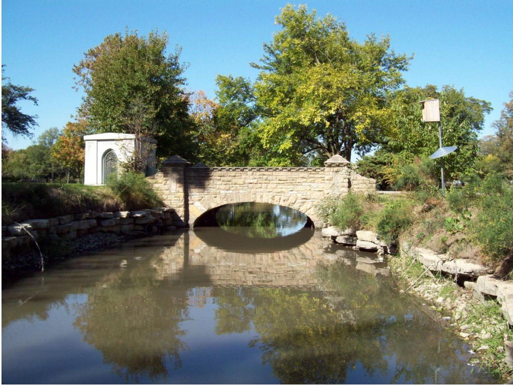
Downstream face of Cemetery Road #1 bridge
