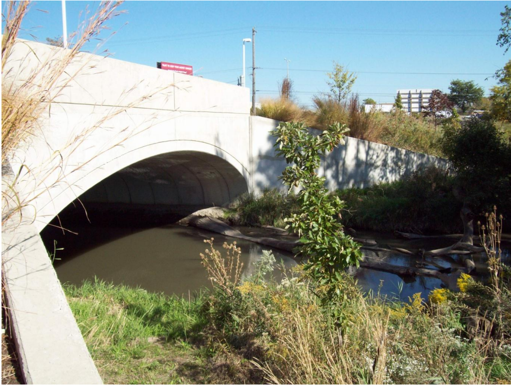
Downstream face of Industrial Access Road from west bank
