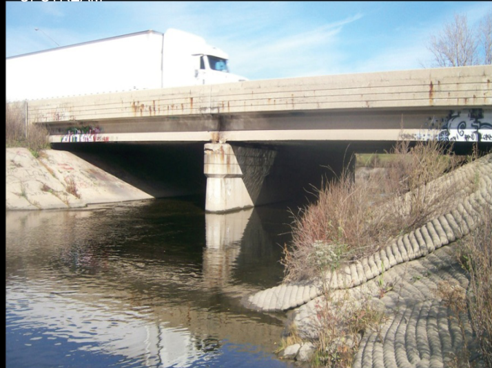
FIGURE 3-21 EXISTING BRIDGE AT I-90 AND HIGGINS CREEK LOOKING UPSTREAM
