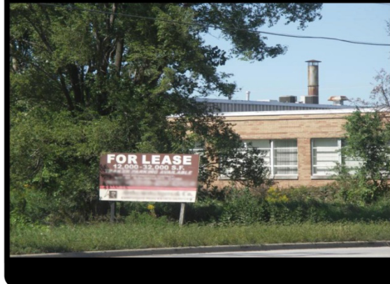
FIGURE 3-3 AGING INFRASTRUCTURE WEST OF O'HARE AIRPORT
