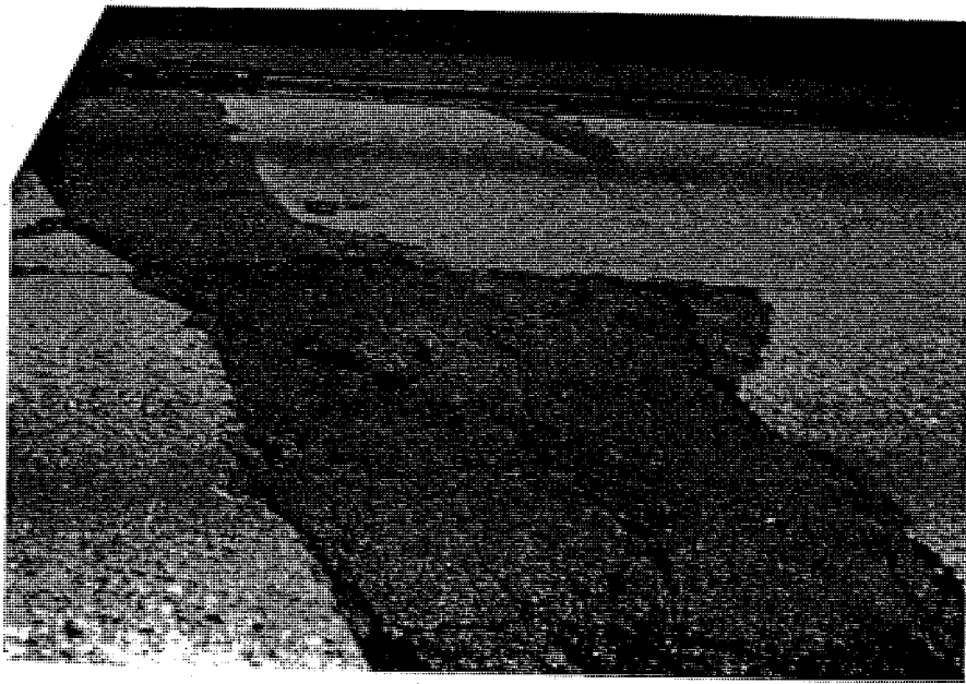
High Severity Asphalt Patch Deterioration
